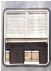
MRVC Window Frame
